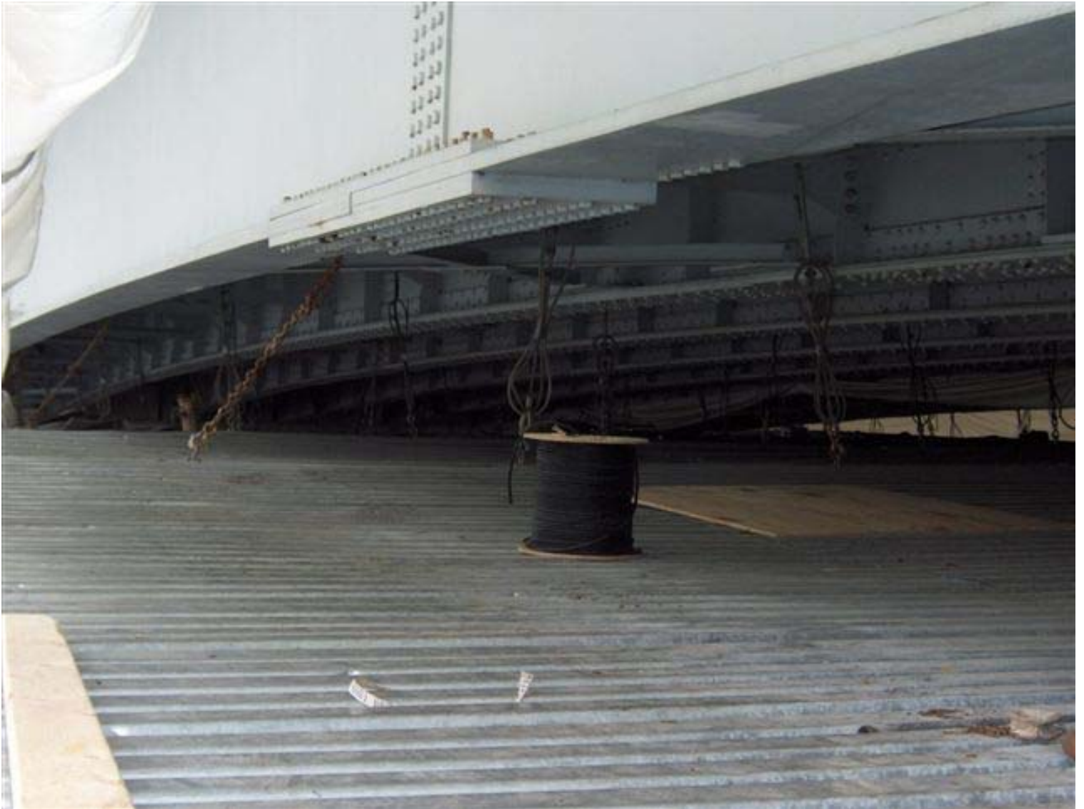
Cable Supported/Metal Deck Platform System
