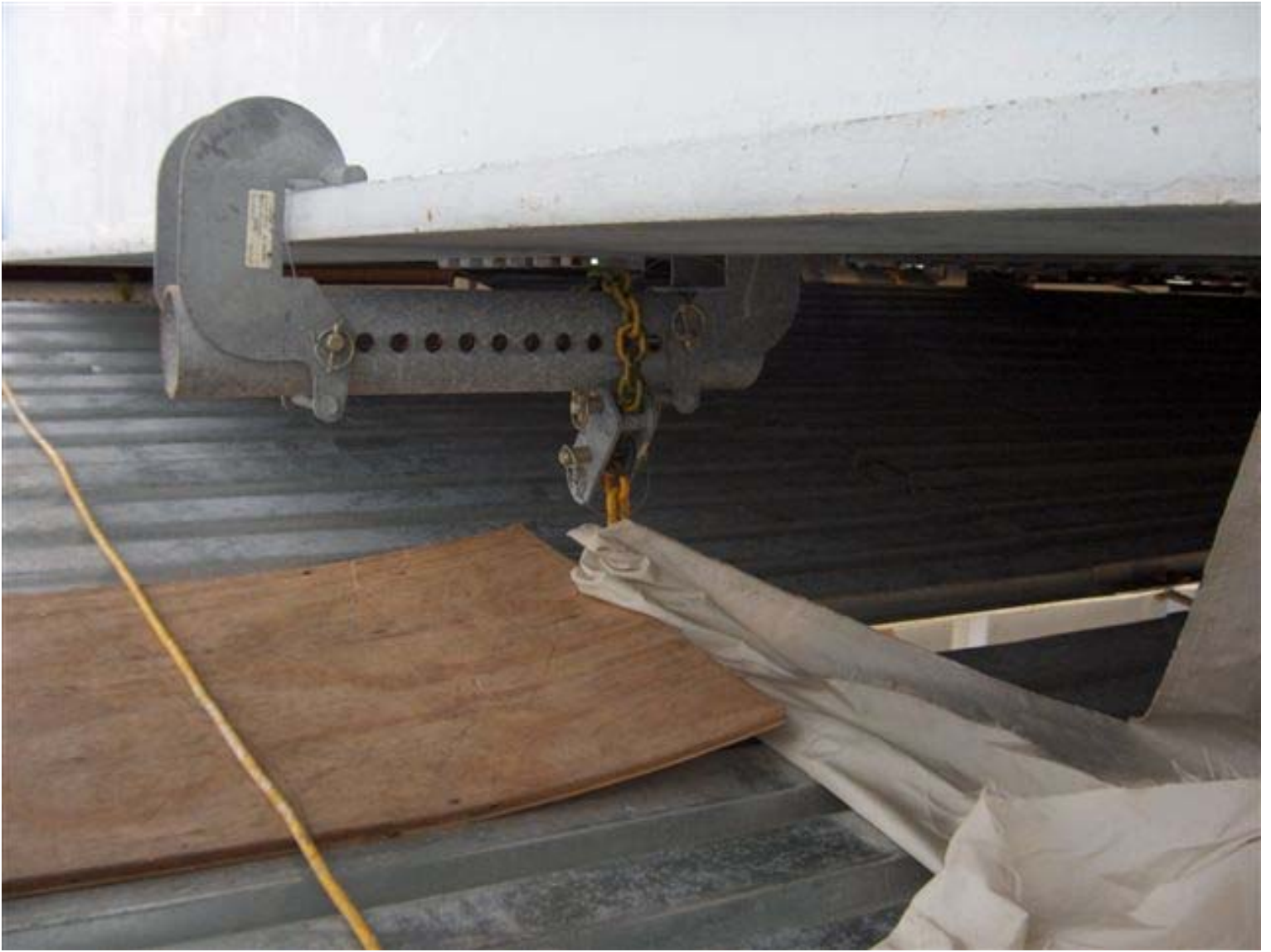
Beam Flange Clamp Hanger Vertical Support
