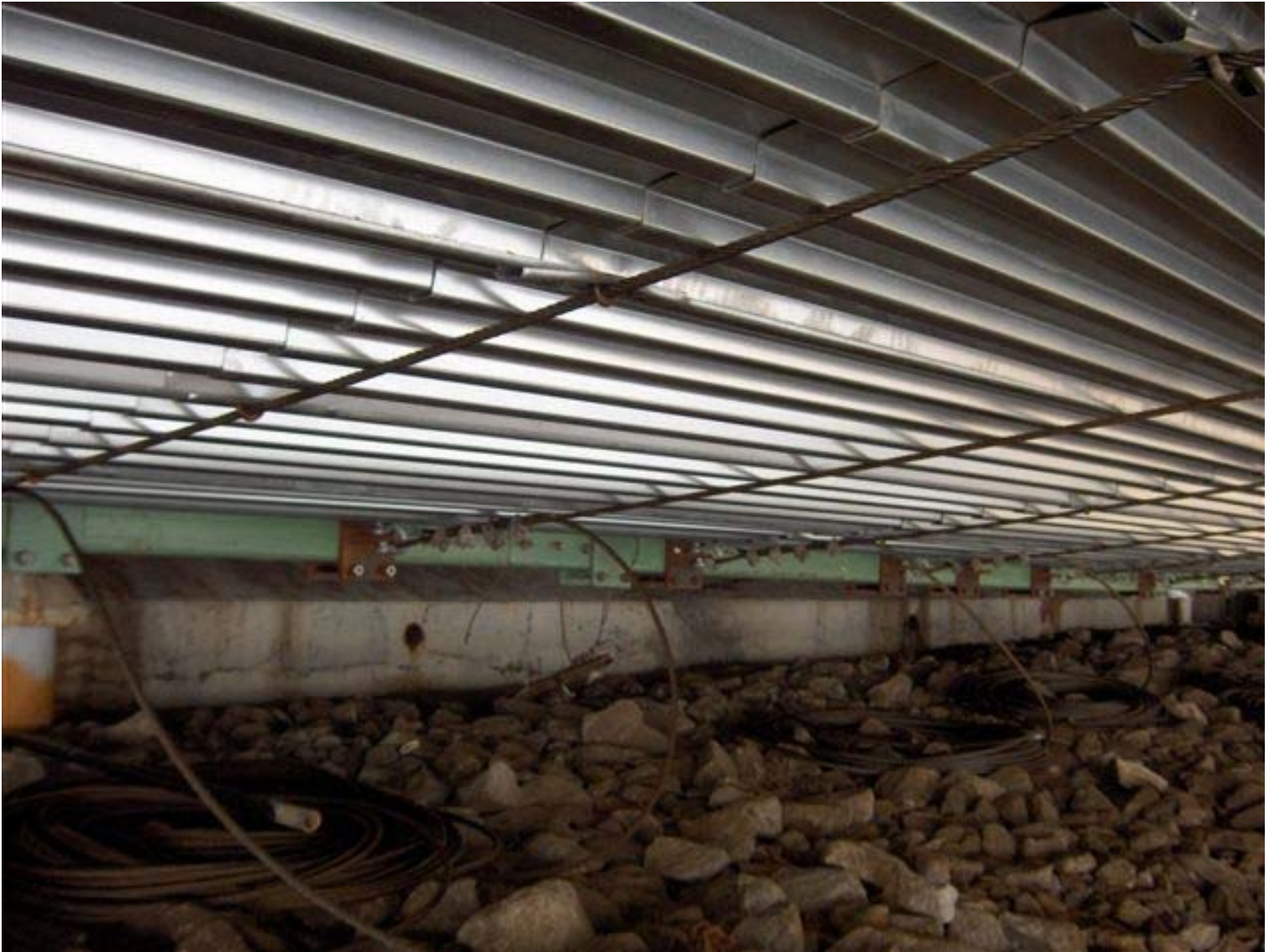
Horizontal End Support Beam Assembly W/Clamping Plate Assemblies For Main Cable Connections
