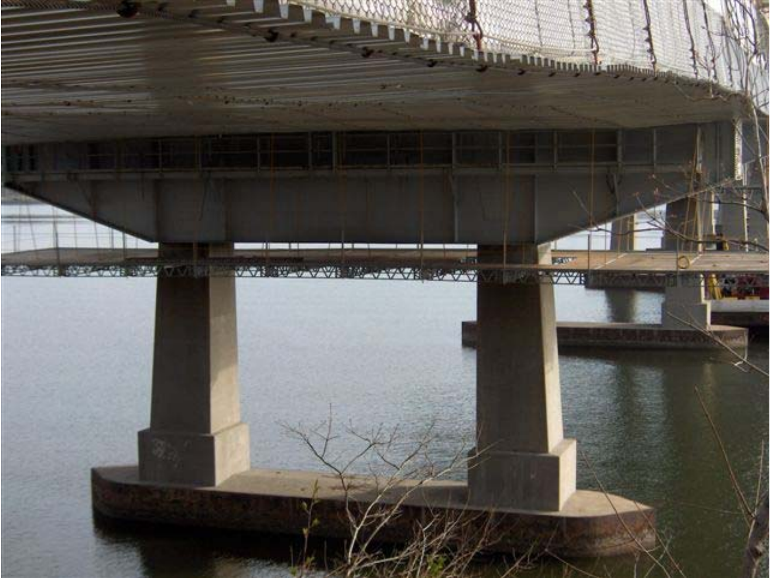
Quik Deck Platform Around Pier Cable Supported/Metal Deck Platform System W/Chain Link Fence Perimeter Protection
