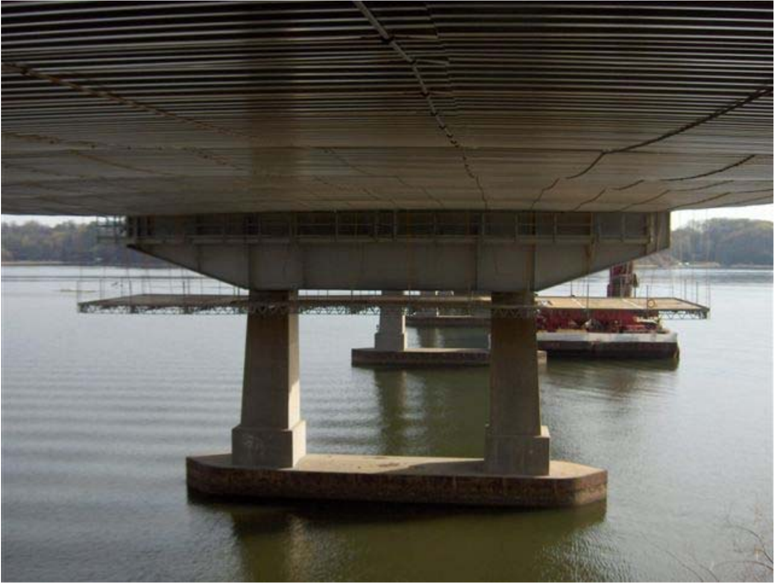
Cable Supported/Metal Deck Platform System
