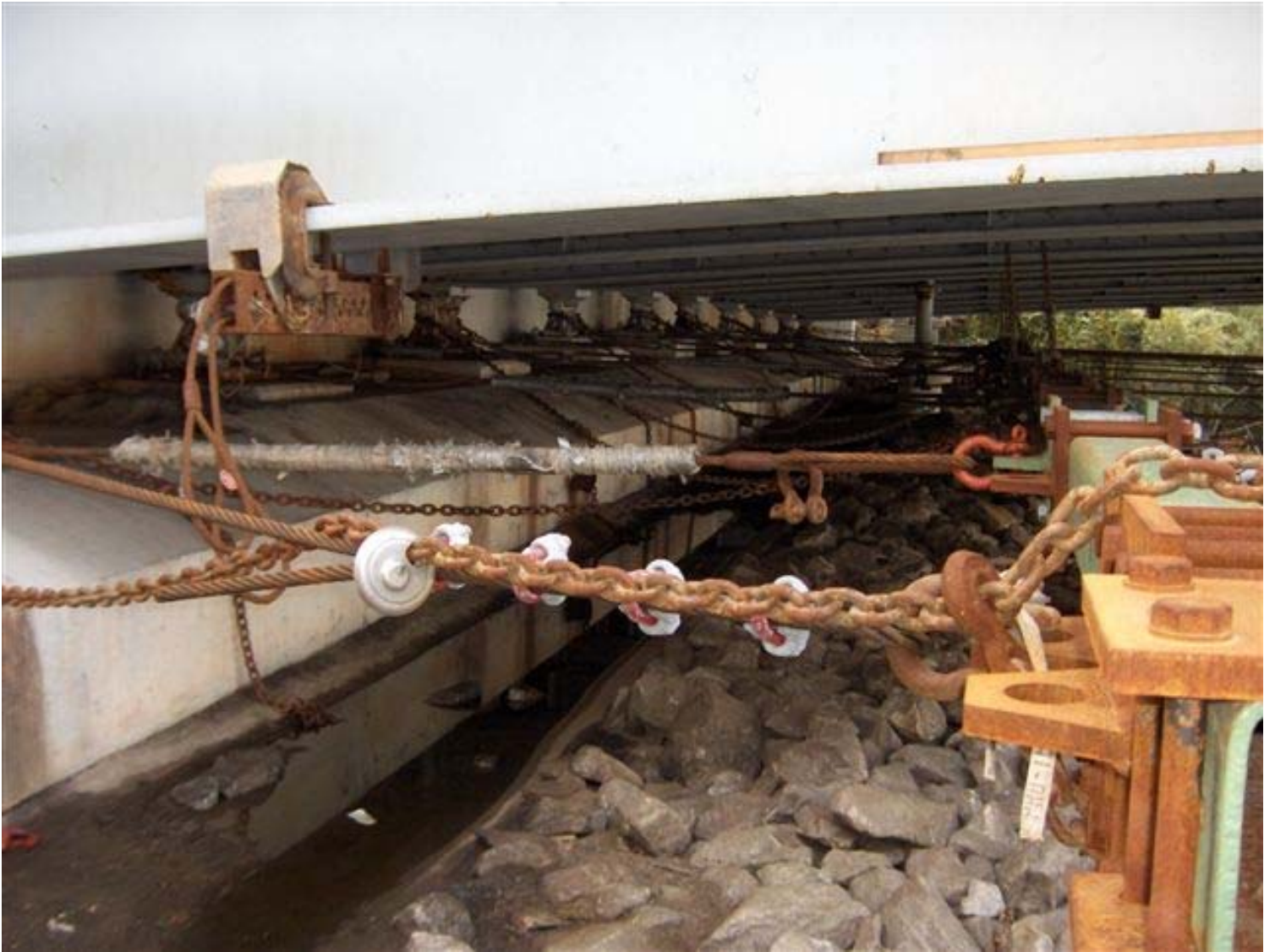
Horizontal Tie Back Assemblies Horizontal Support Beam To Bridge Bearings
