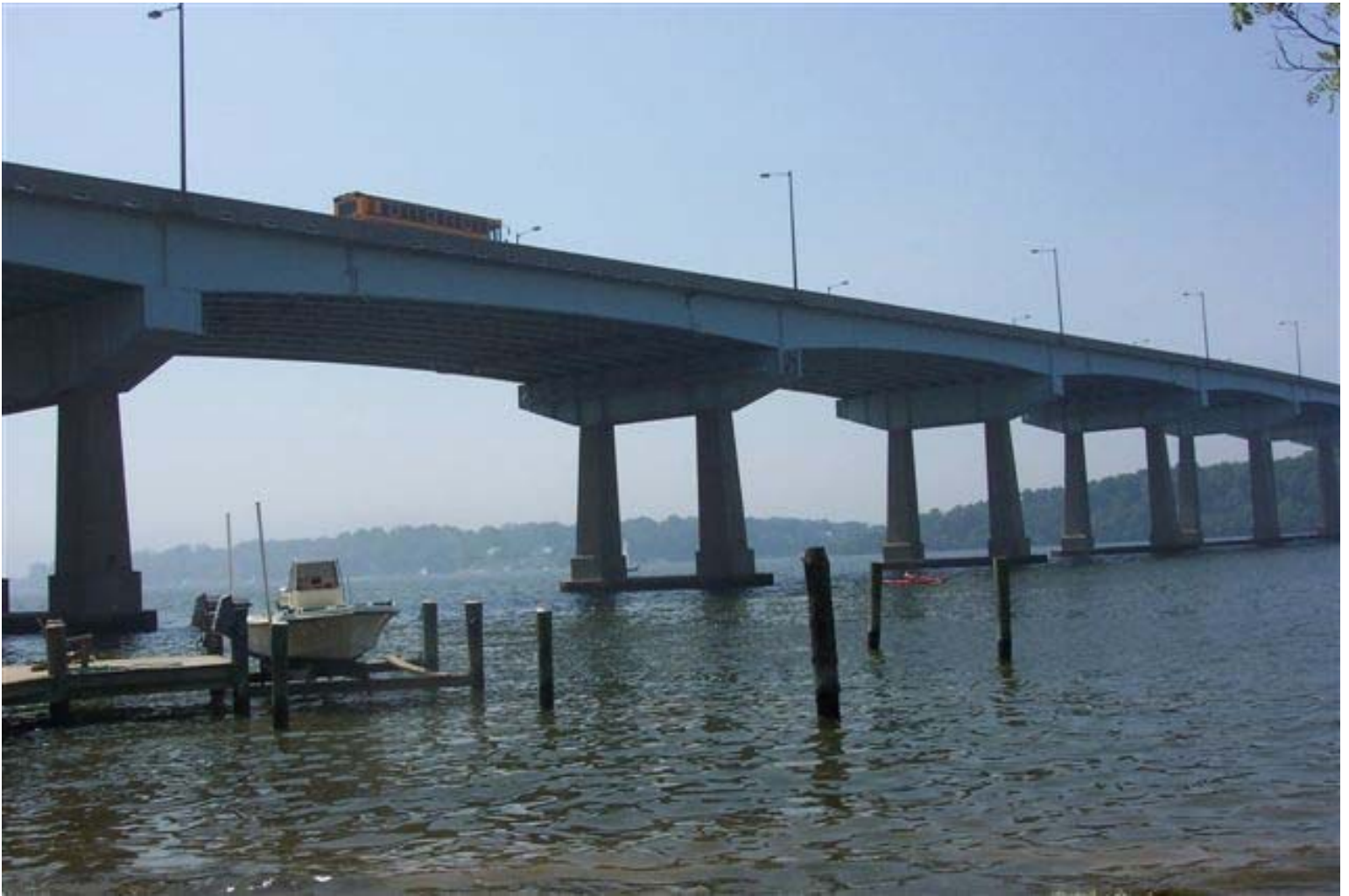
17 Span Girder Bridge (US Rte. 50) Over The Severn River
